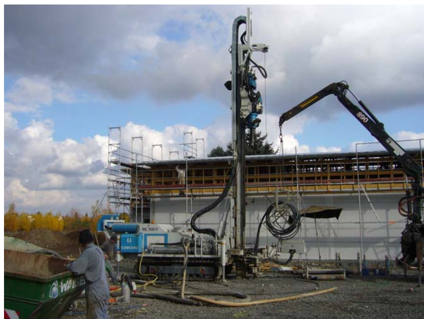
Figure 3: Drilling for a supermarket BHE project in Western Germany
